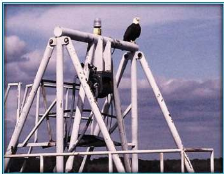
Figure 4: Bald Eagle Perching on the Mast of the Anchor Barge
