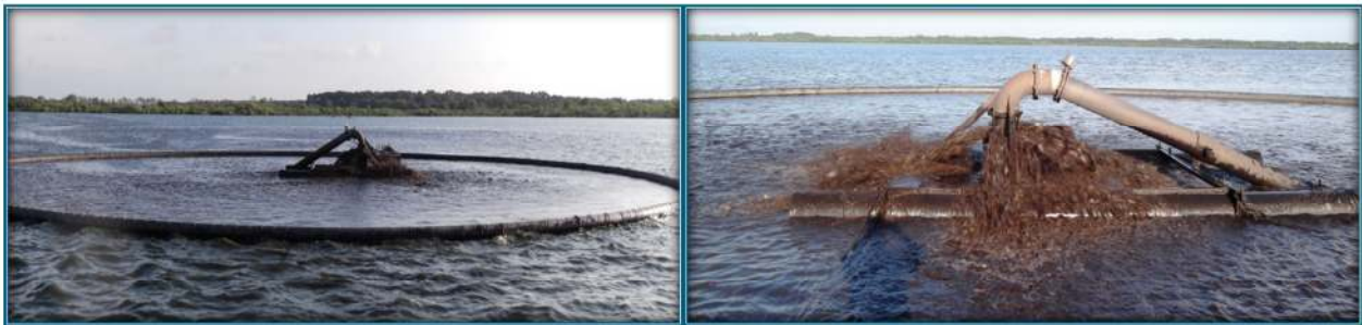
Figure 2 and 3: Jahna Dredging Disposal Ring control Turbidity and Deposition Levels along with Aerating Discharge Water
